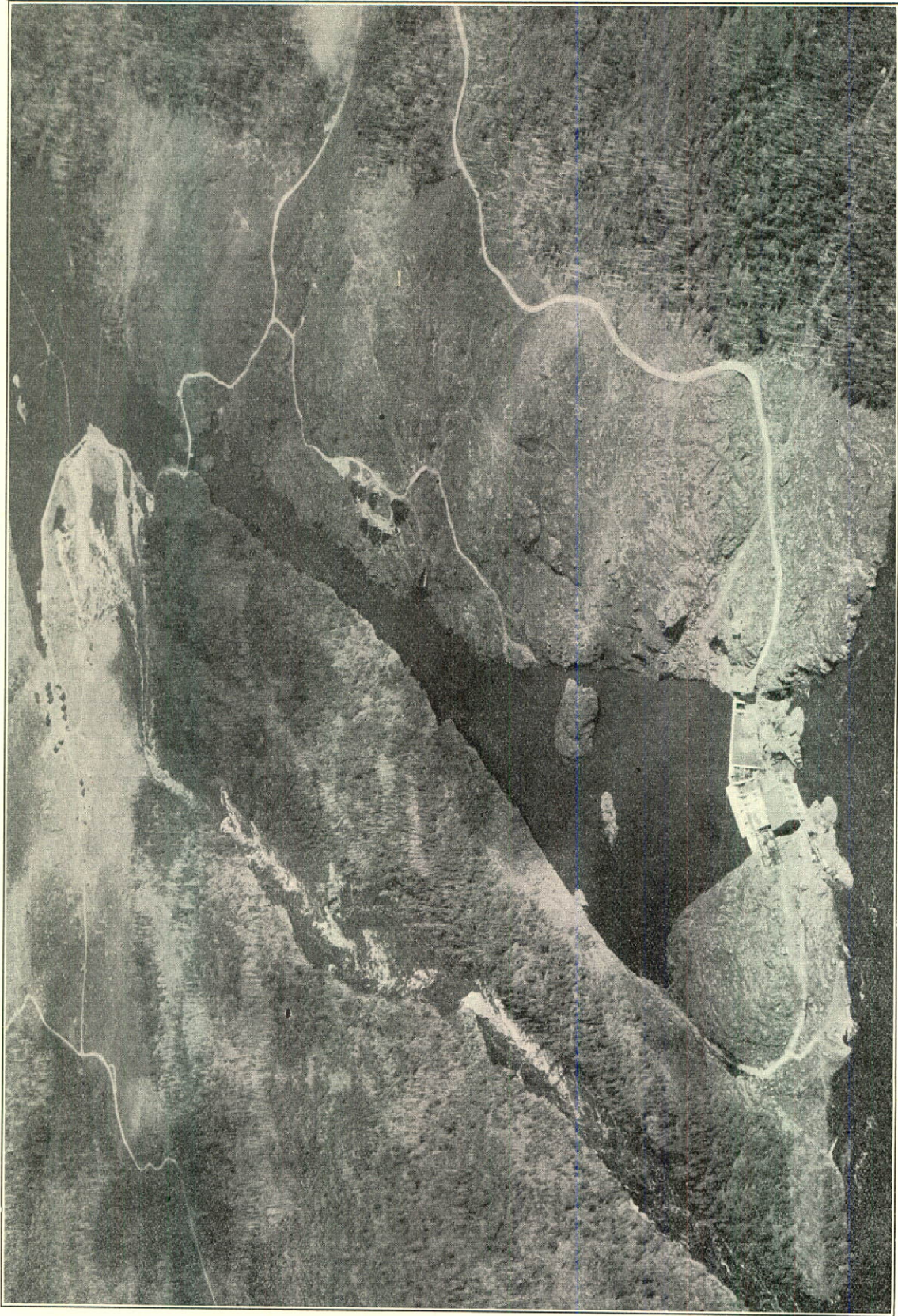
Aeroplane view of Quinze Power Plant—Two additional Units now being added
