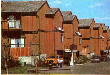
Mortgage loan insurance provided under the National Housing Act gives Canadians improved access to housing appropriate to their needs.
