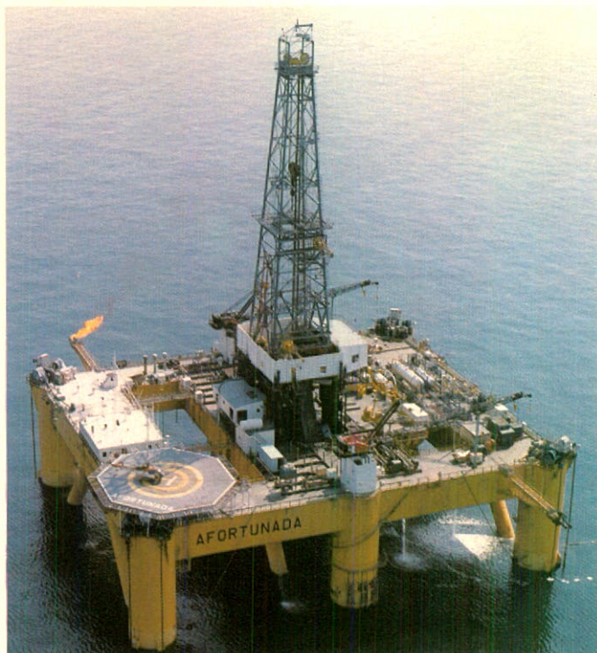
The Afortunada on location with the Casa 1-A well on production in a drill stem test mode and the Casa 6 well producing through a Colflex-ip (flexible flowline) riser to the production facilities located on the aft deck of the Afortunada (left of the derrick).
