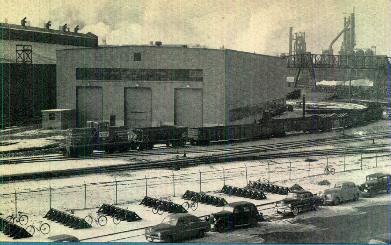
New Diesel Electric Maintenance Building for servicing thirteen new diesel electric locomotives
