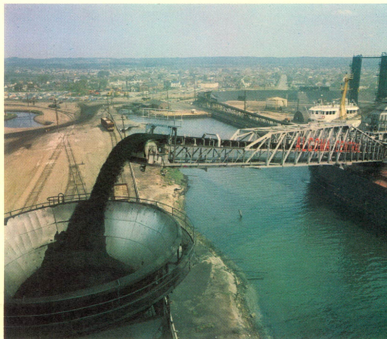
Coal is shipped to the Steelworks in self-unloading vessels.
