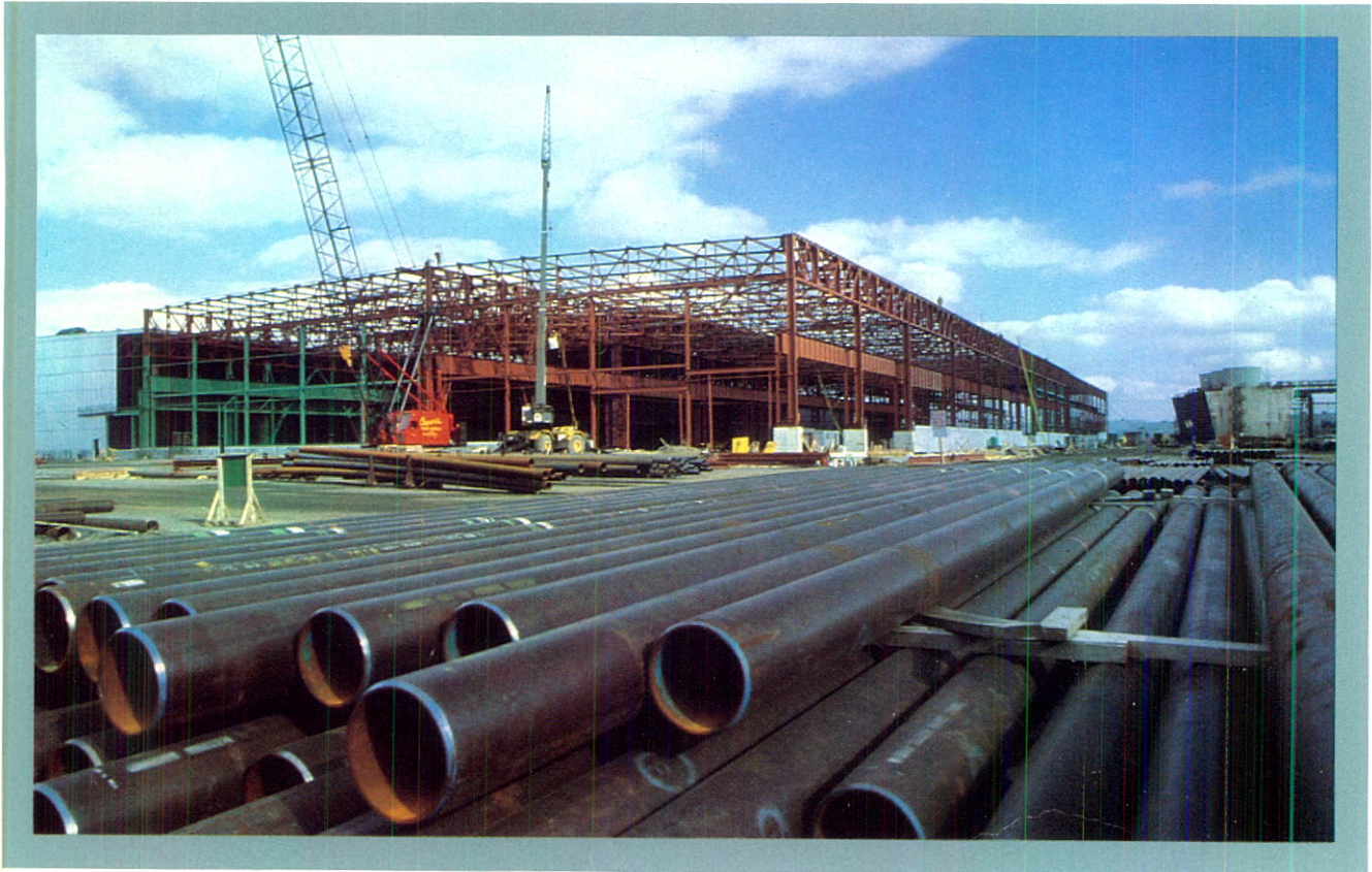
New seamless tube mill under construction.
