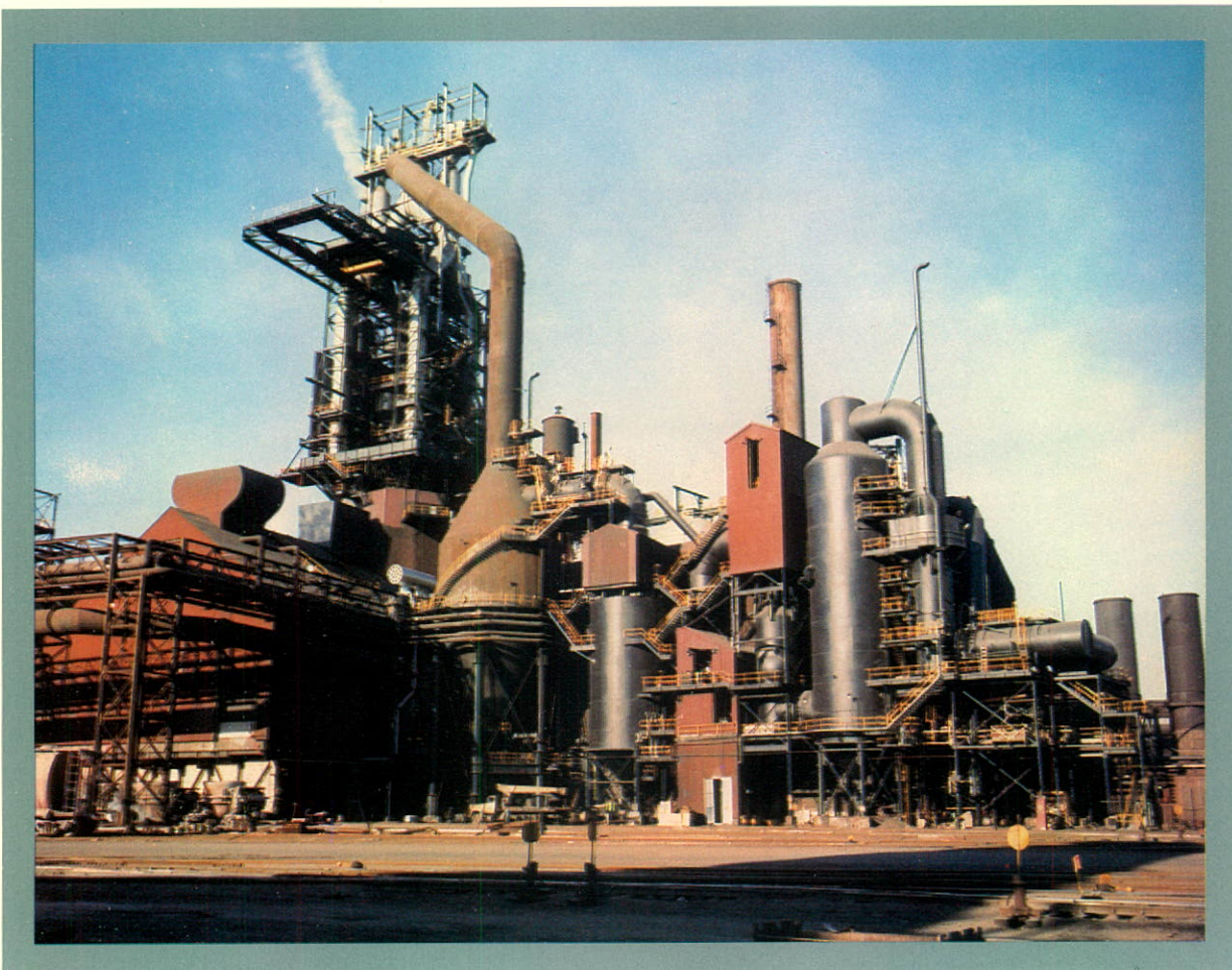
No. 7 blast furnace was relined and modernized in 1981.
