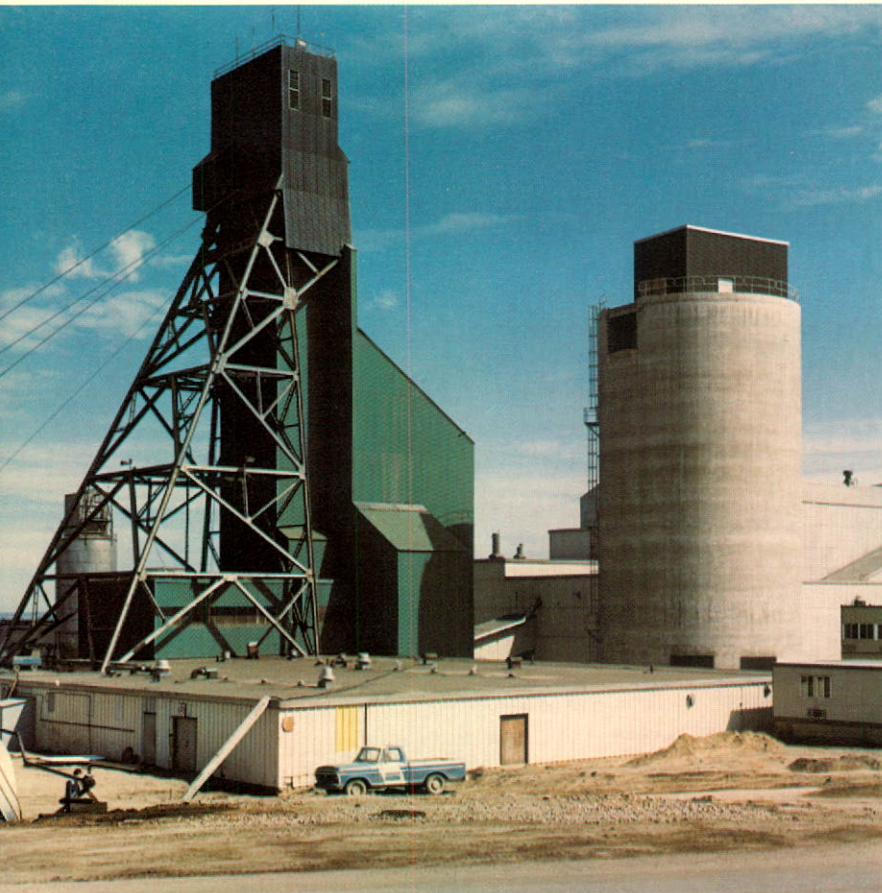
No. 2 headframe and new ore bin
