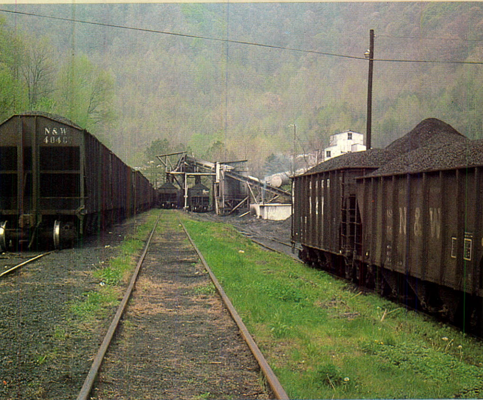
Railcar loading facilities at the preparation plant. The siding can accommodate 22 loaded cars and is adjacent to the N & W rail line.
