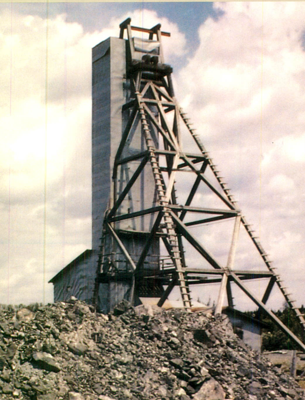
Headframe constructed in 1972 as part of an underground program to provide bulk samples for pilot plant tests.
