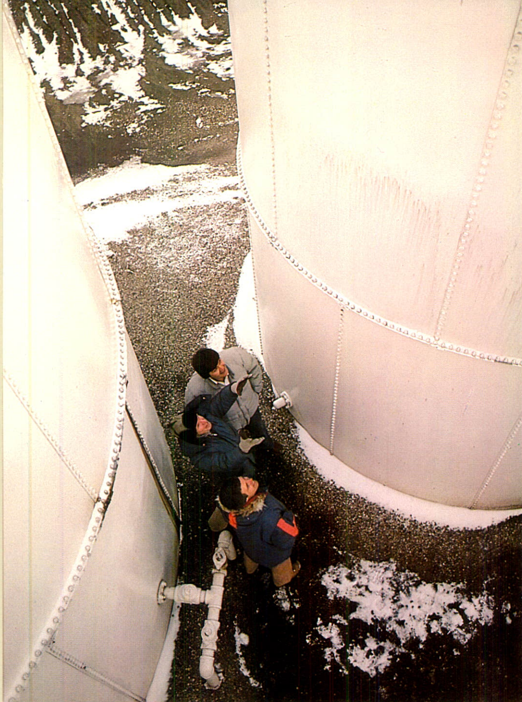
Mike Huculak, Steve Clement and Wayne Jessee viewing field installations.
