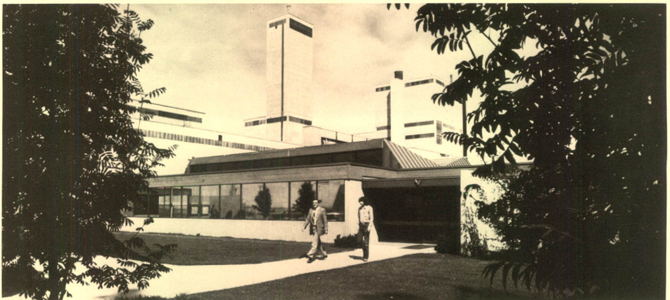
Cariboo Pulp & Paper at Quesnel, B.C. is virtually energy self-sufficient.
