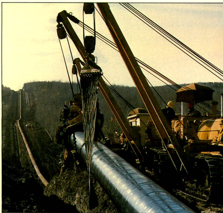
Wrapping and coating 36-inch pipe in a looping project.
