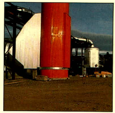
The Company's new processing plant at Pine River as it neared completion in mid-1979. Above, thermal oxidizer unit at bottom of the stack incinerates waste gases and minimizes the emission of impurities into the atmosphere.
