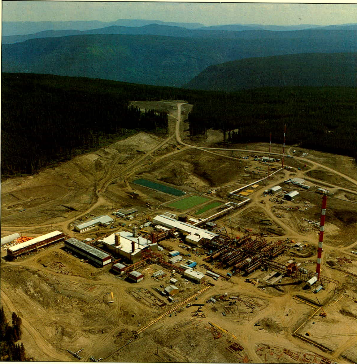
The Company's new processing plant at Pine River as it neared completion in mid-1979. Above, thermal oxidizer unit at bottom of the stack incinerates waste gases and minimizes the emission of impurities into the atmosphere.
