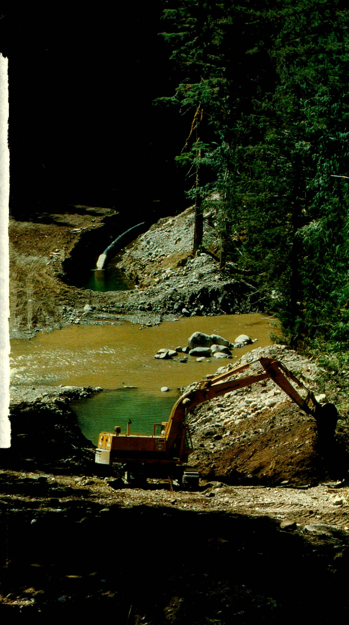
Crossing the Coquihalla River with 36-inch diameter pipe. All such river crossings are supervised by fish and wildlife authorities to assure habitat protection. Above, the river after the pipe is buried in riverbed.
