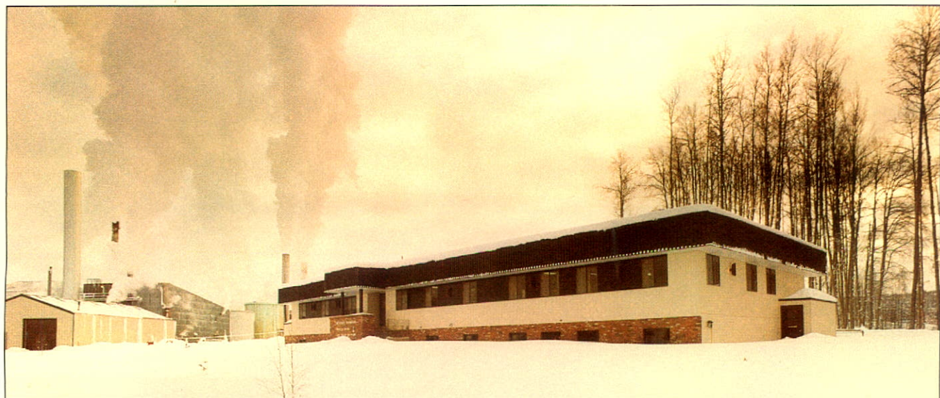
New Office — Fort Nelson Gas Processing Plant
