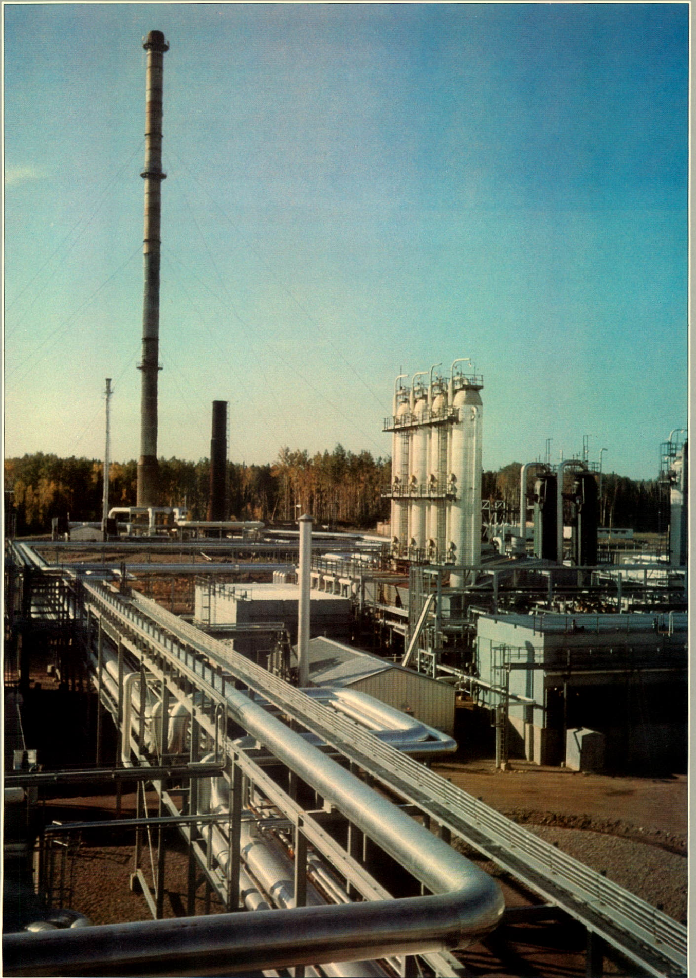
Fort Nelson Gas Processing Plant
