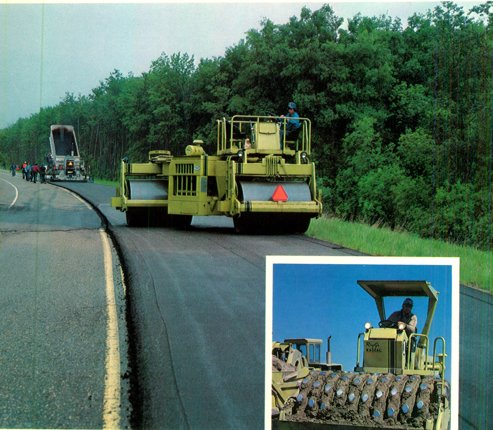
(Large photo) RayGo Ranger 2-66 compactor. Rolling asphalt on a provincial highway near Daulphin, Manitoba.
