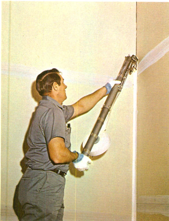
Taping drywall with Ames tool
