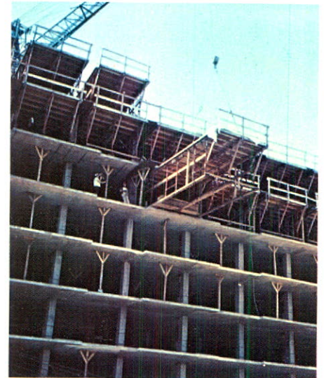
Apartment complex, Washington, D.C.
