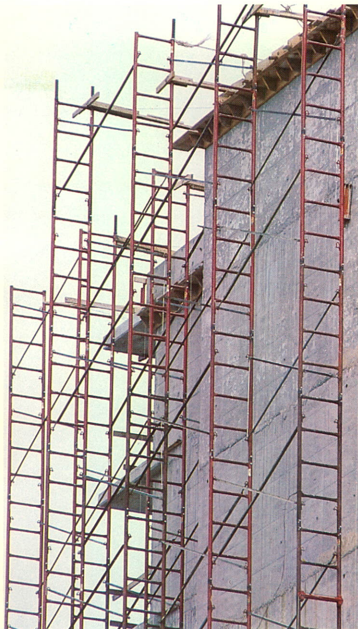
High rise construction—Waco scaffolding
