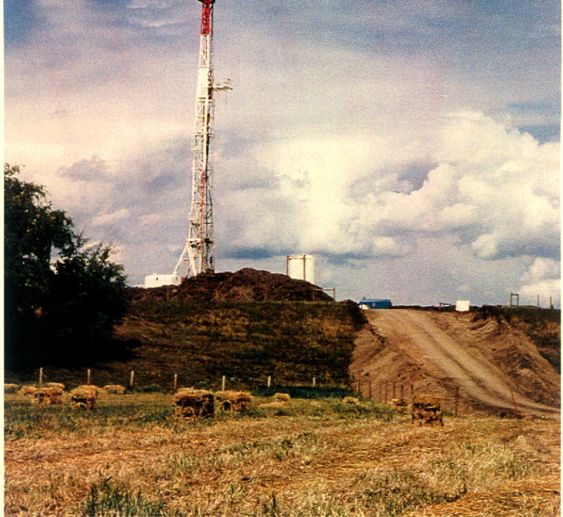
Drilling Rig, Ponoka area.
