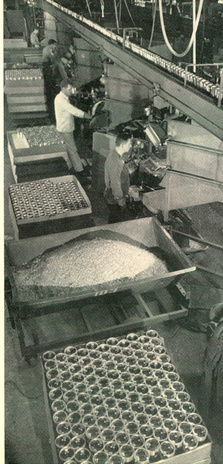
Rough turning and inspection of pistons
