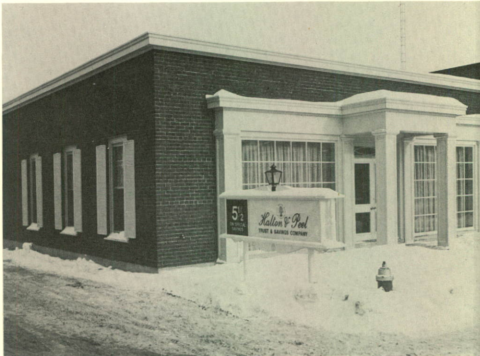
Latest addition to Canada Trust—Huron & Erie branch system, an office was opened in Kitchener's Stanley Park Plaza late in 1968. It features the distinctive "sand-dollar" decor. (BELOW) Attractive office of Halton & Peel in Georgetown is ideally adapted to its surroundings. It was built in 1966.
