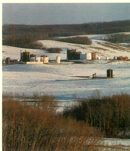
Cleaning plant and truck pit terminal at Tangleflags, north-east of Lloydminster.
