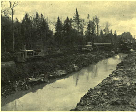
Big inch pipeline stringing operation in Northern Ontario.
