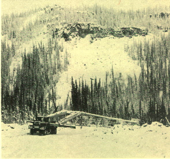
Moving a derrick to a drilling location within the Arctic Circle (outside temperature -58 degrees).
