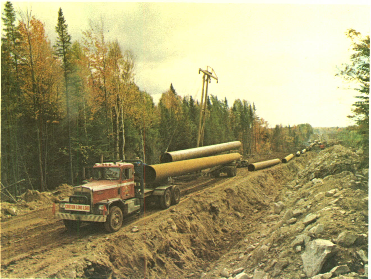
Pipeline stringing in Northern Ontario for 36" looping program.
