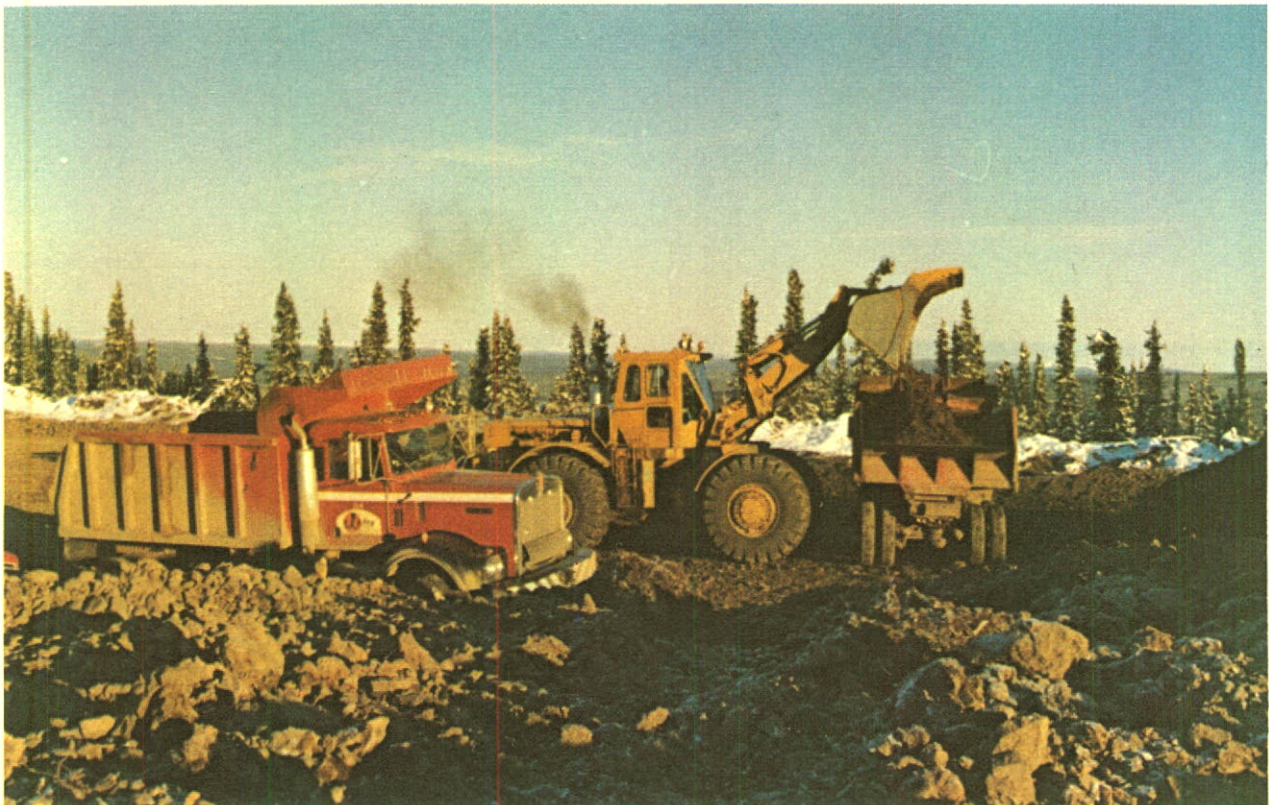
One of the large front end loaders in the process of loading a dump truck at one of the active borrow pits on the Dempster Highway.
