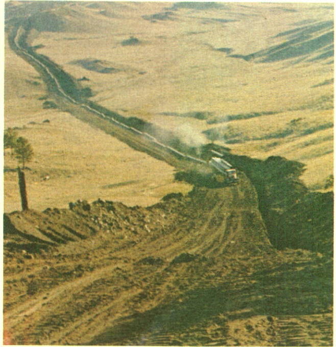
Portion of a pipeline stringing job in Montana, U.S.A.
