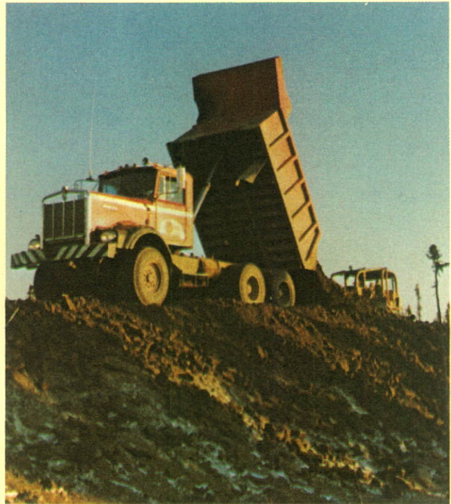
Equipment engaged in building the road bed for the Dempster Highway project.
