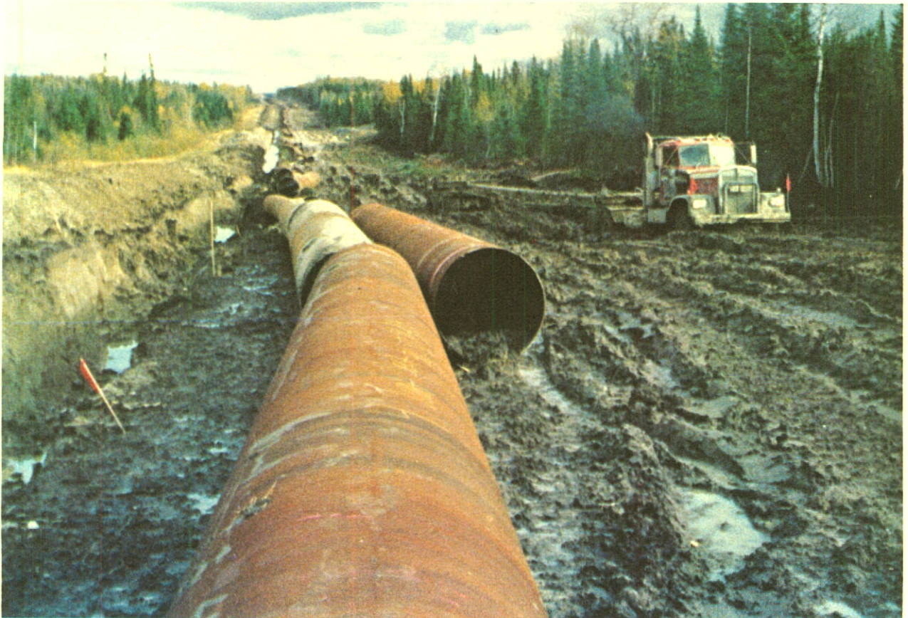
Typical pipeline right of way during the summer months in Northern Ontario.
