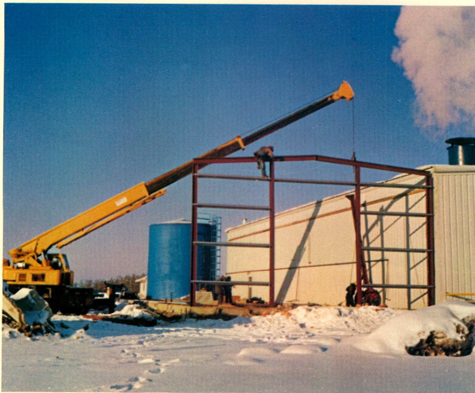
Berth for Thermo II, 1979 Phase II Expansion
