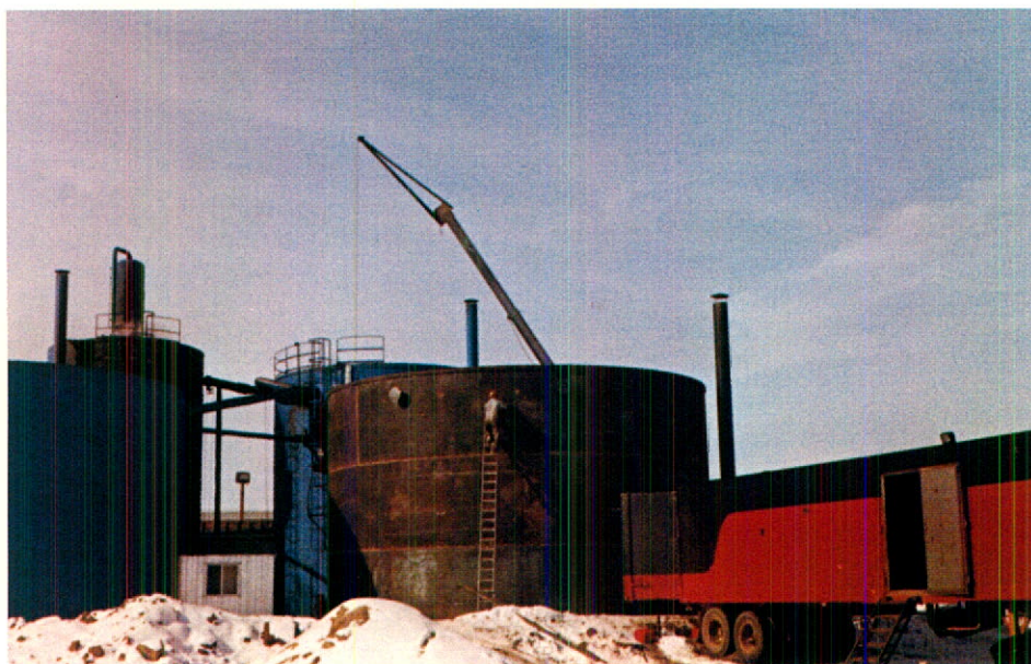
Additional 5,000 bbl. storage tank for Phase II Expansion
