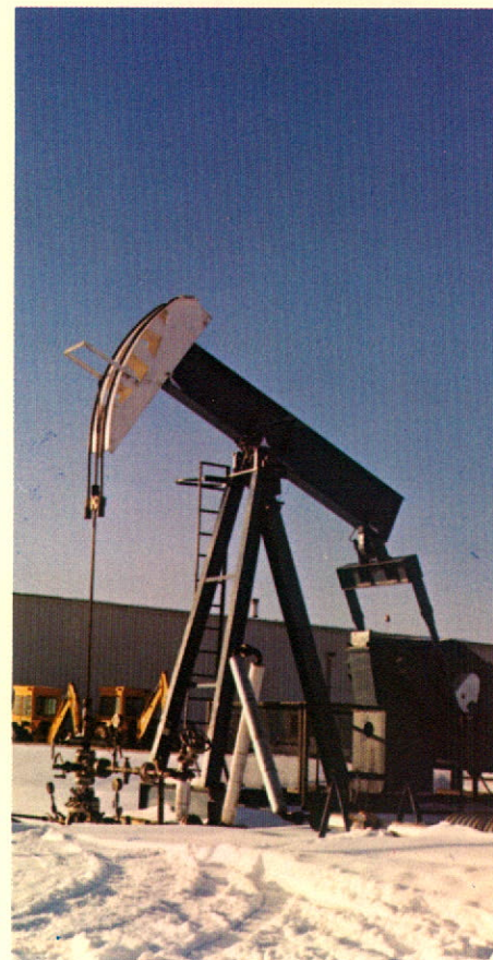
Producing well close to steam building.
