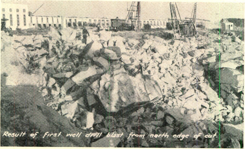
Seven Sisters Falls: Showing quantity of rock displaced by one blast.
