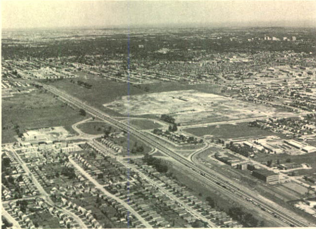
Aerial view of Yorkdale site as construction commenced in 1962.
