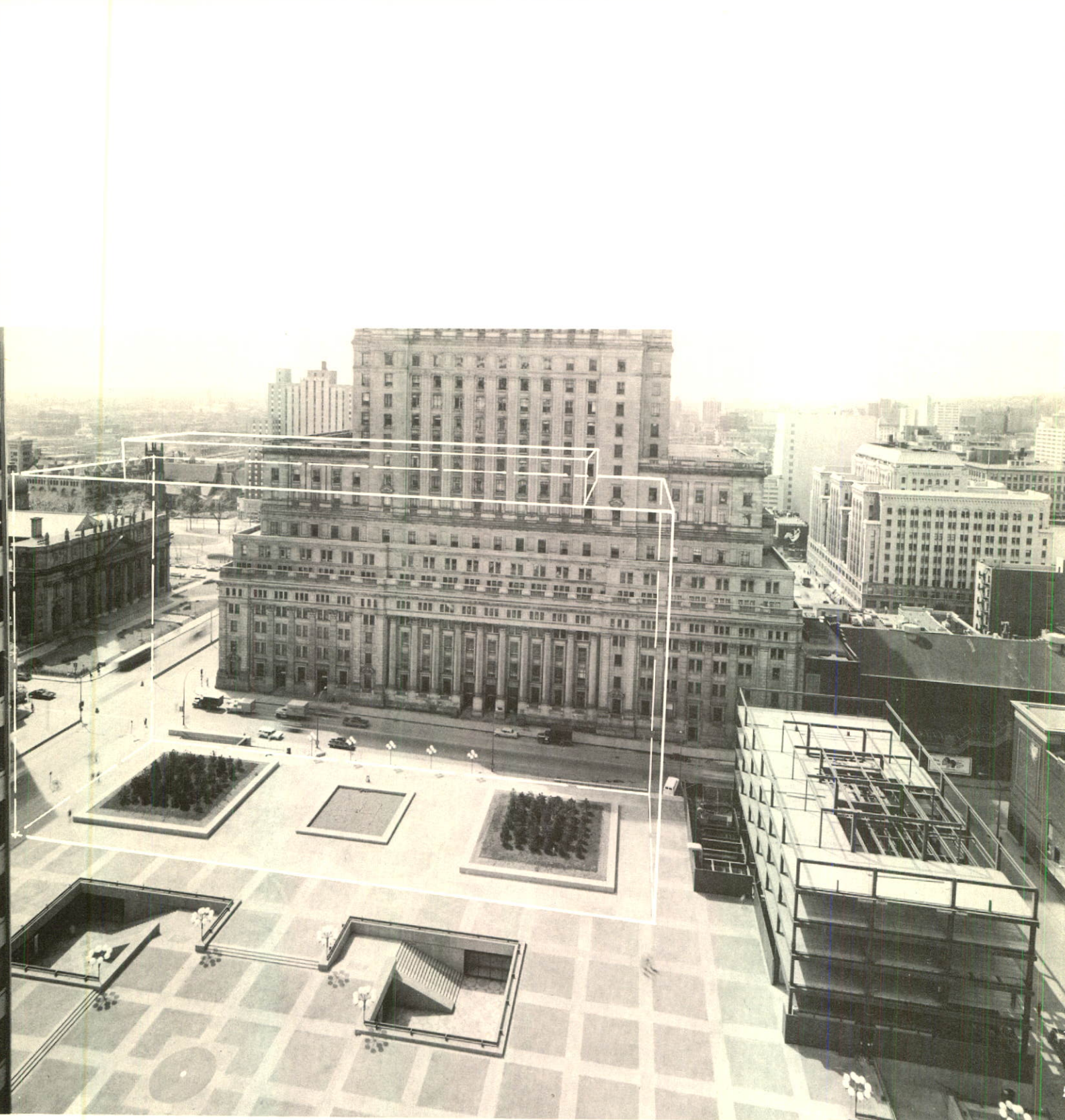
Place Ville Marie Plaza showing Greenshield House under construction and the site of the remaining building.
