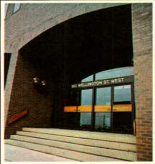
180 Wellington Street West Building, Toronto
