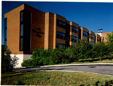
Albion Road Nursing Home Toronto, Ontario
