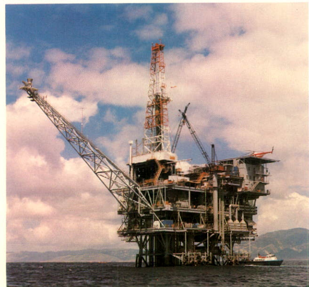
22,000 foot capacity platform rig, drilling off the coast of California.
