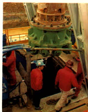
Large diameter shaft rig drilling in Manitoba.
