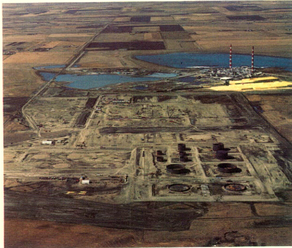
Refinery Construction Site — Calgary, Alberta
