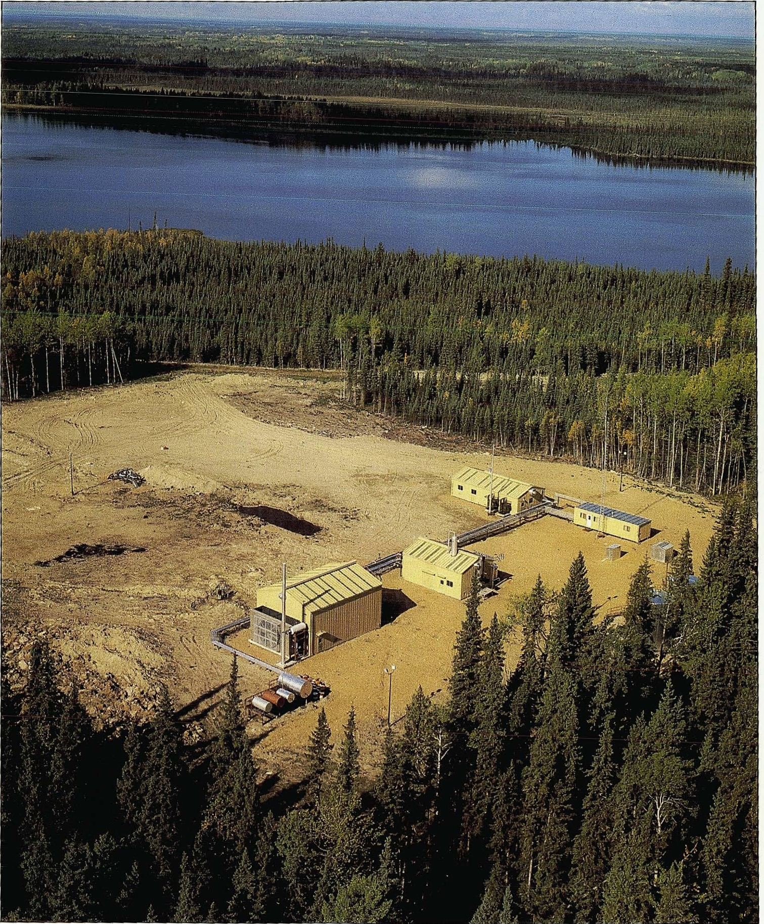
Gas plant at Clyde
