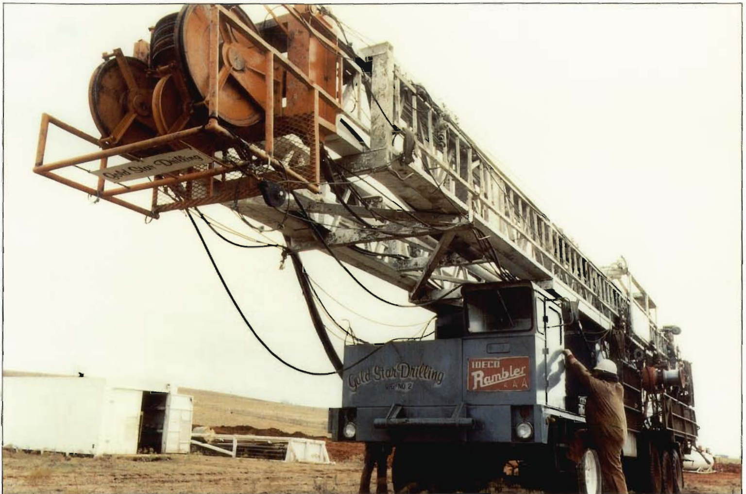
Relocating a Gold Star rig
