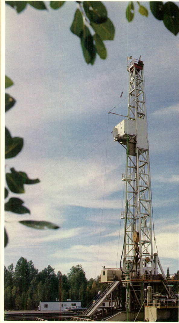
Drilling in the Karr area, south of Grande Prairie, Alberta.
