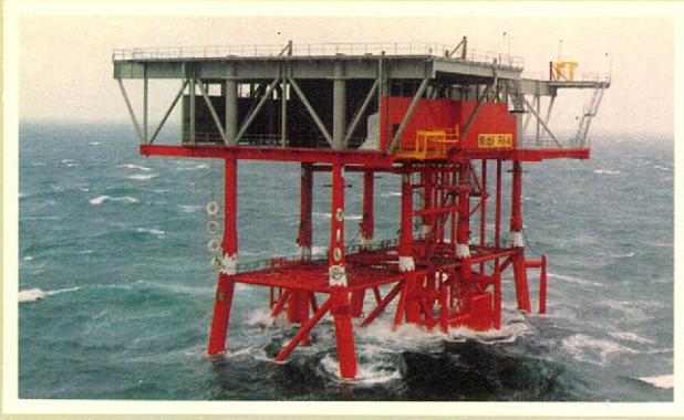
Production platform jacket and deck in the offshore Netherlands Block P/6 gas field.
