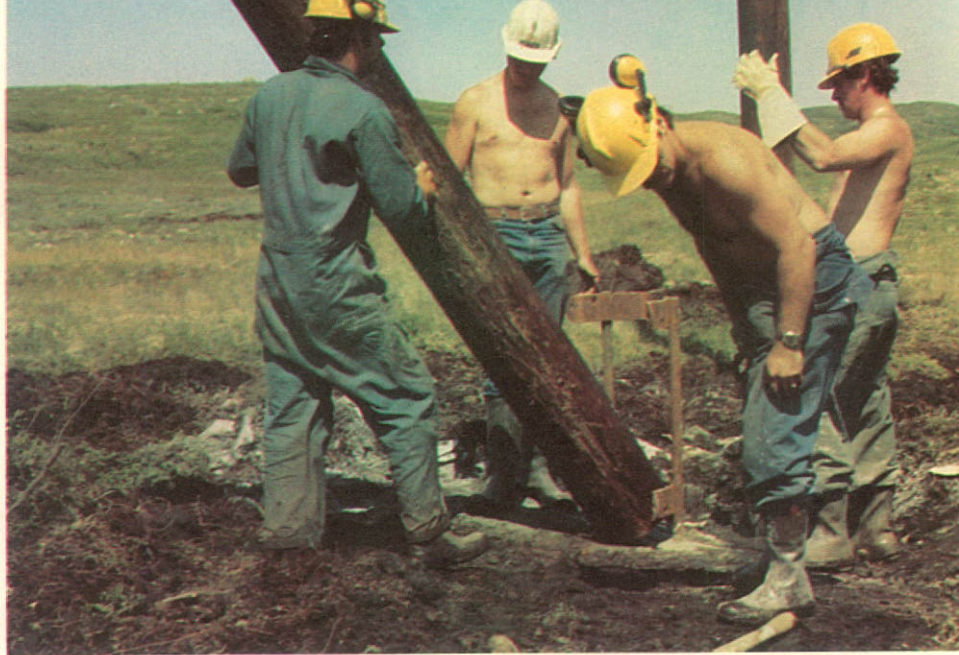
An innovative "rock-mount", designed to solve pole erection problems across extremely rocky terrain.
