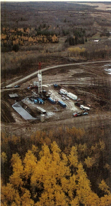
Lindbergh site in early stages of construction
