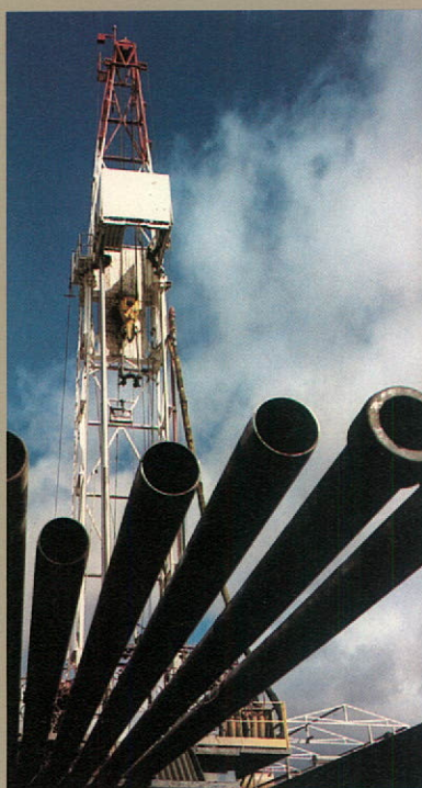
Drilling operation, Lindbergh
