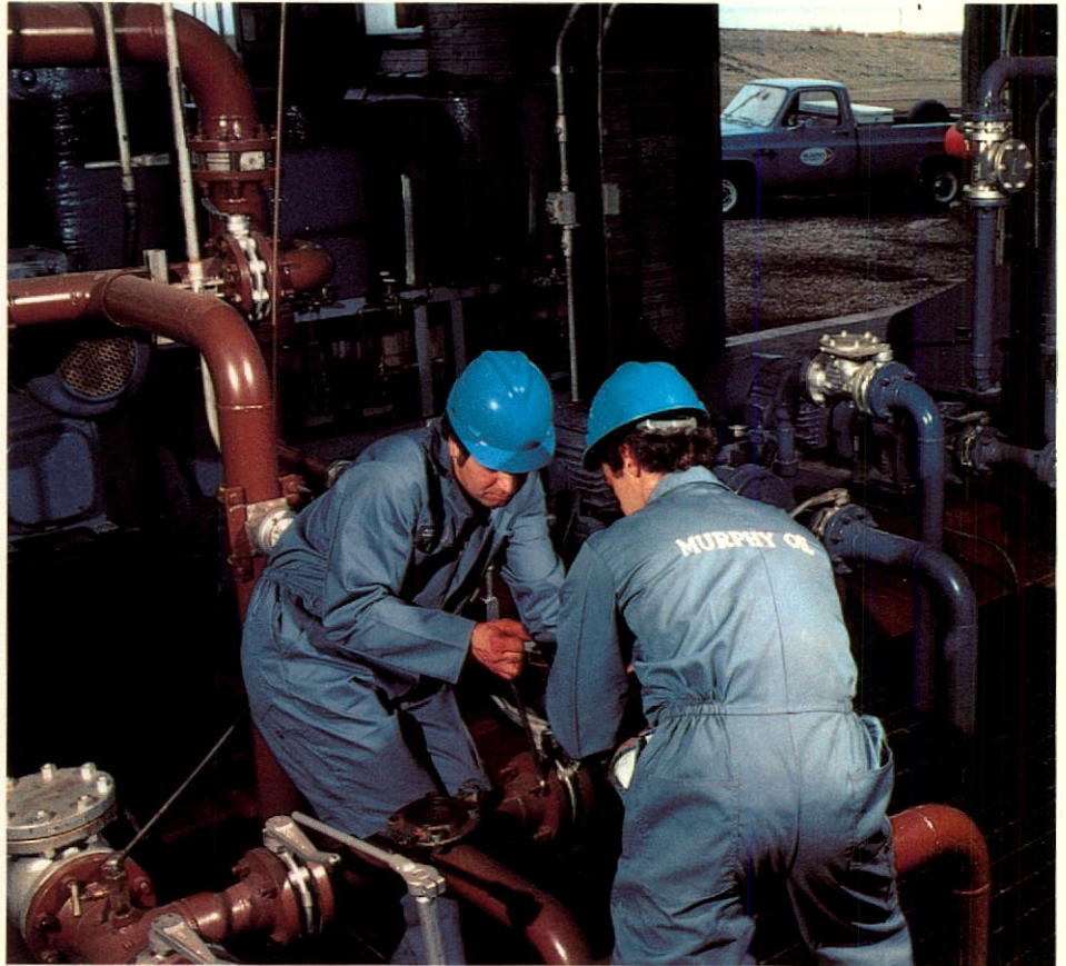
Maintenance at treating plant, Eyehill Thermal Recovery Project.
