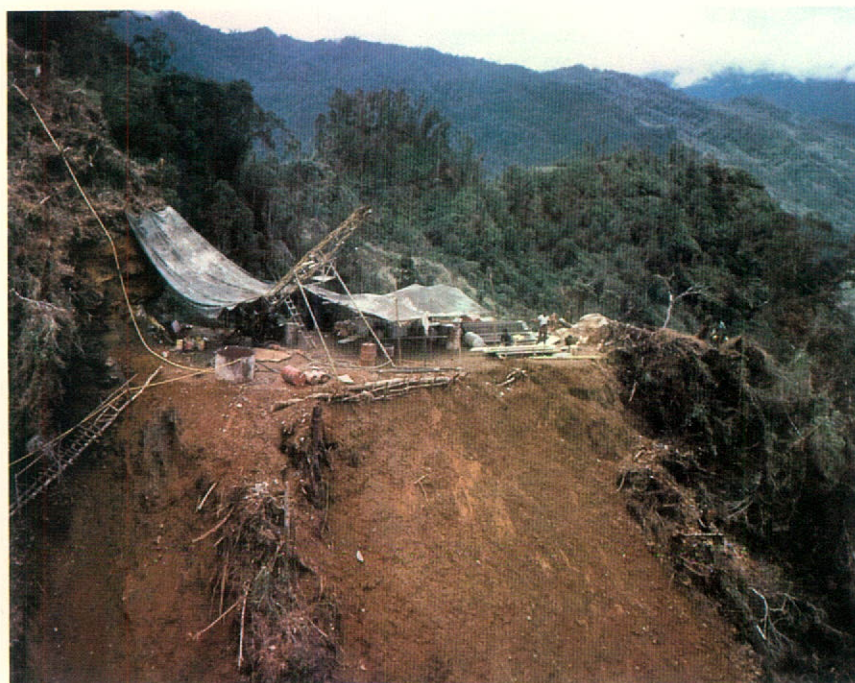
Exploration for gold was continued at Misima and Porgera in Papua, New Guinea. At Porgera, numerous drill pads similar to the one shown, were built with pick and shovel to allow diamond drilling on the mountain slope.
