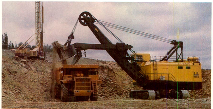
Ore for the Equity mill is loaded, while drill prepares another bench for production blast.
