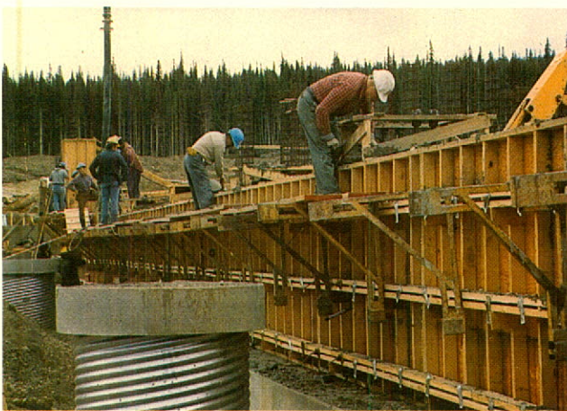
A – Foundations for the concentrator building are poured during a summer drizzle. B – Finishing the concrete before removing forms. Ore will be ground and concentrated in this building before passing to the leach plant. C – Rain gear is an important item of equipment.
