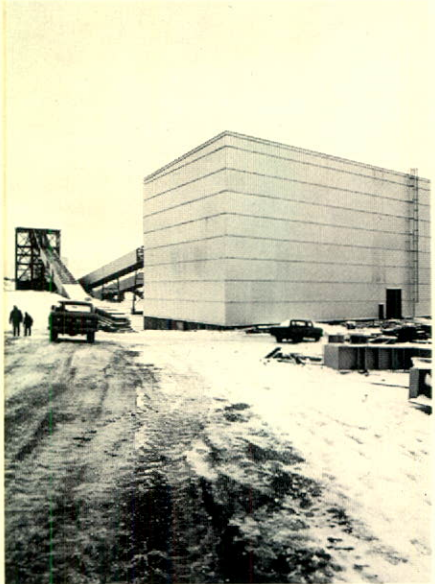
Secondary crusher building and conveyors.
