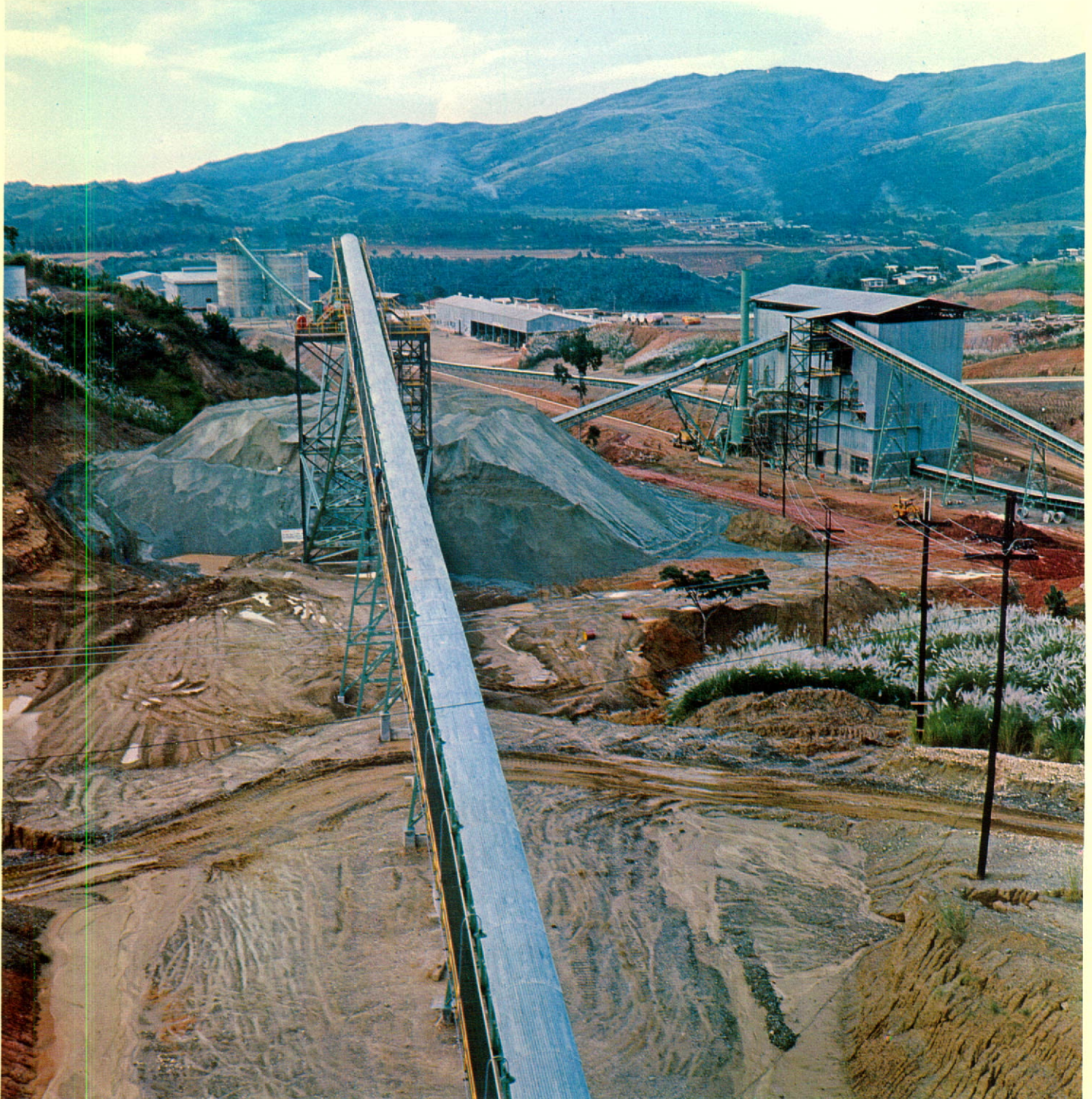
A view of the Marcopper operation from the primary crusher showing the secondary crusher, workshops, fine ore bins and the process water tank.
