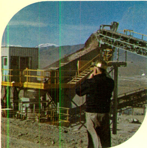
A view of the conveyor belt at Cortez.
