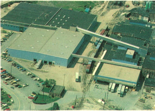
Interfolded absorbent paper towels (left) are among the many products made at the new manufacturing and storage facility (above) at Berlin, New Hampshire.
