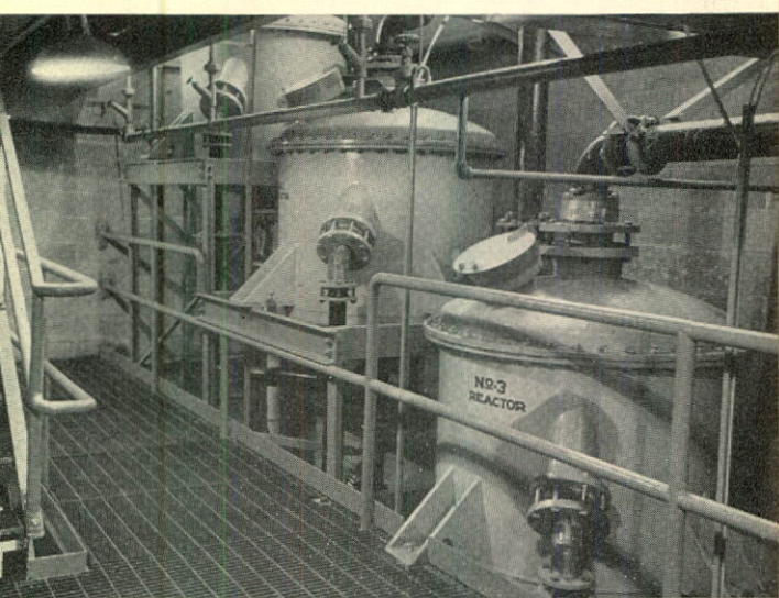
Chlorine dioxide reactors, installed in the new \text{ClO}_2 plant, are part of the equipment necessary for the chain of chemical reactions required.
