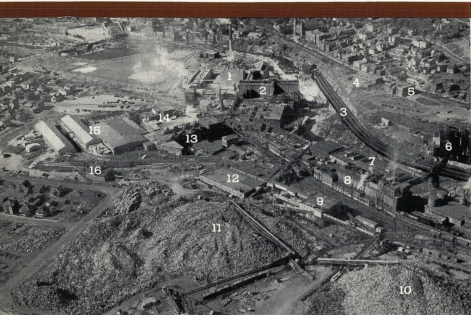
A portion of Brown Company's concentration of plants at Berlin, N. H. Individual units are: 1 — Kraft pulp mill; 2 — Burgess sulphite pulp mill group; 3 — Penstocks carrying water to Riverside power house; 4 — Woods and Personnel departments; 5 — Administration building; 6 — Portion of Bermico tube mill; 7 — Riverside paper mill;
