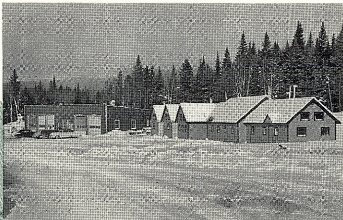
▲ A typical installation in Brown Company woods is this new garage and camp at Long Pond, Maine, on the new forest road built by the company to open up the Parmachenee region.
