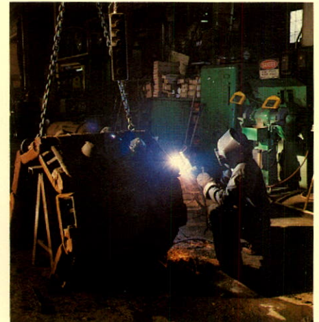
Depositing alloy metals to restore worn areas of huge mining shovel track pads used in Quebec mines.
