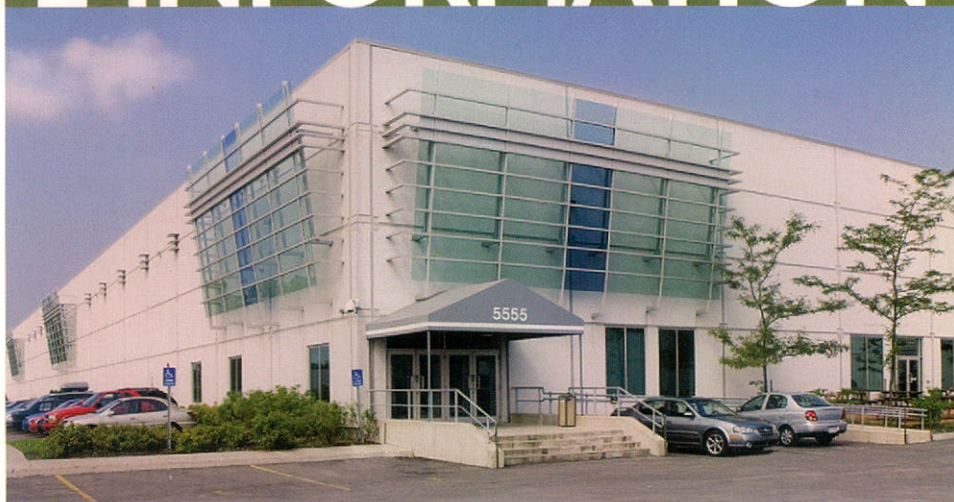
Reitmans Distribution Centre, Montreal, Québec
