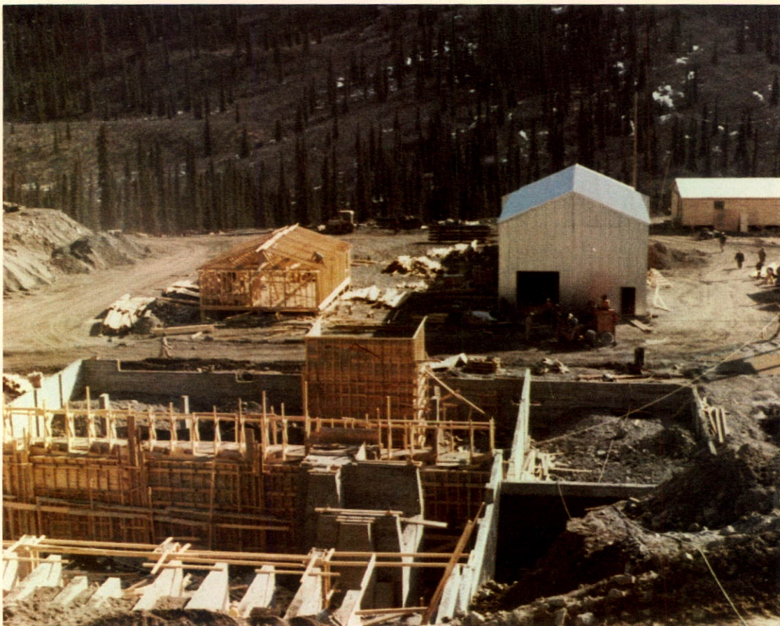
Mill and powerhouse in early stages of construction.
