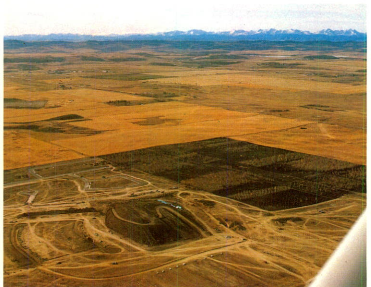
Canada Trust and Costain Limited are developing this 446 acre site in southwest Calgary. Plans call for over 2,000 housing units plus commercial and industrial lots. Servicing of phases one and two will be complete in early 1981.
