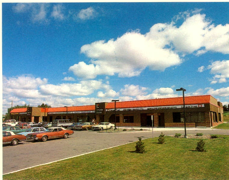
Lincoln Plaza, well-located on one of the busiest suburban streets in Waterloo, Ontario, was acquired in 1978 and completely renovated in 1980. A Canada Trust financial services branch and real estate office are among the tenants.
