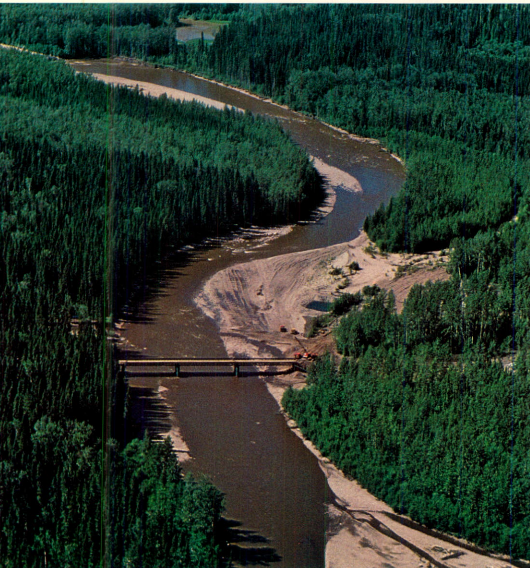
Bridge constructed over the La Biche River assures year round supplies for the Kotaneelee field on all-weather highway leading from Liard River staging area.
