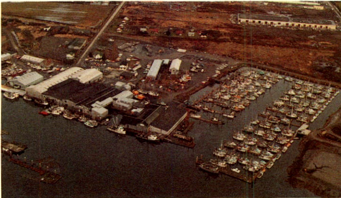
Aerial view of Boat Basin and service area, rebuilt and enlarged during 1977.
