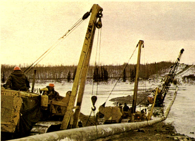
Wonderly & Kershaw installing a pipeline across the North Saskatchewan River
