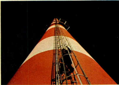
Sulphur compound monitoring system on an Alberta gas plant stack
