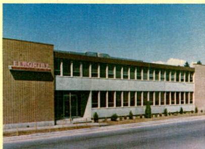
Elworthy's new office addition in Vancouver
